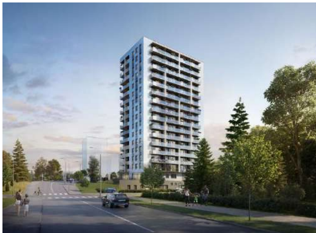
SkyHome @Infra group
